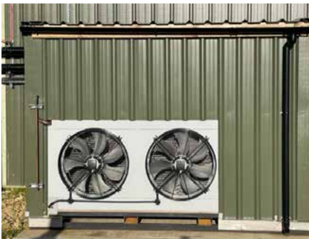
Figure 4: Plant room exterior
